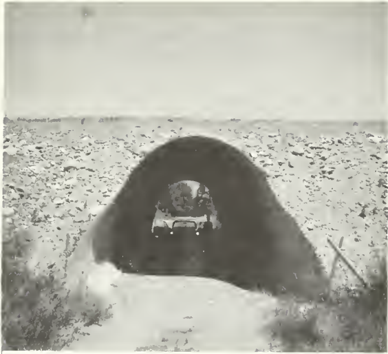
SOUTH ENTRANCE looking North
